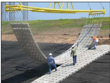
flexible cellular concrete mat
