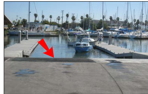
vertical curve at head-of-ramp
