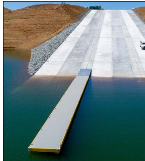
cable-guided boarding float
