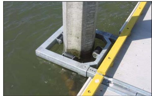
exterior pile yoke
