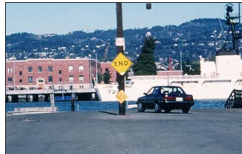
boat launching ramp with safety warning signs: at end of access road, and at top of launching ramp
