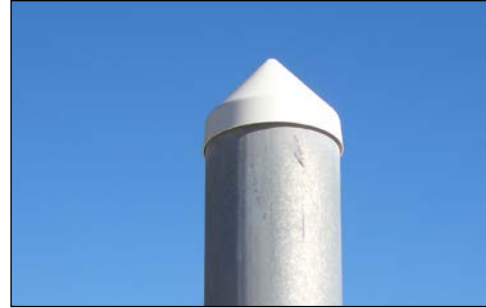
guide pile with “cone” cap
