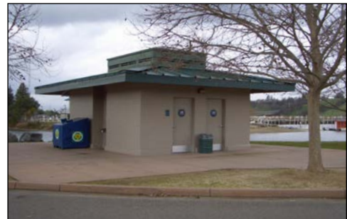
restroom at boat launching facility
