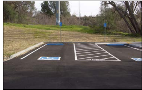
parking space markings. note accessible aisle border should be blue color
