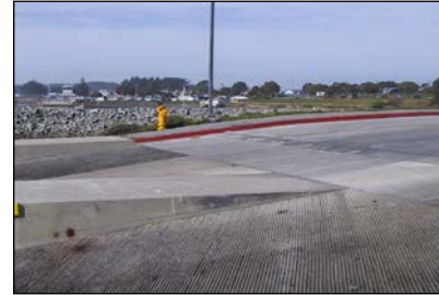
boarding float abutment
