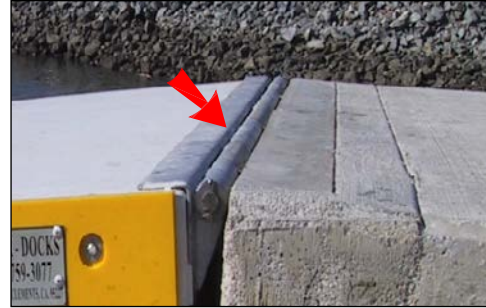
boarding float-abutment hinge
