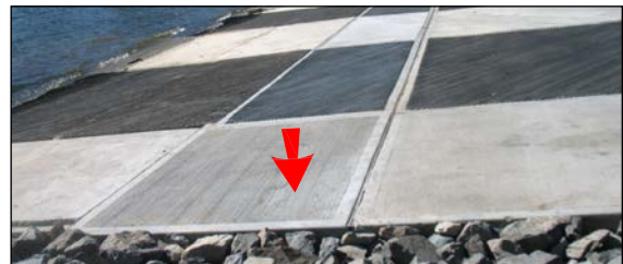
completed closure section
