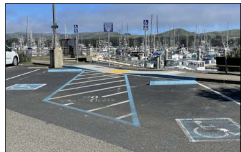
accessible ramp and access aisle
