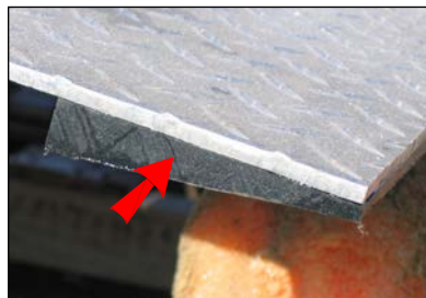
6 inch gangplank wearstrip wedge
