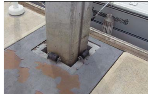
square concrete guide pile
