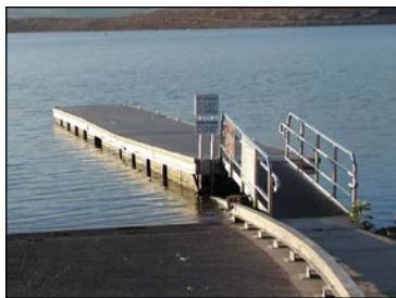
single-rail steel beam guided boarding float
