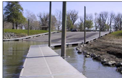
external guide piles along outside edge of floats
