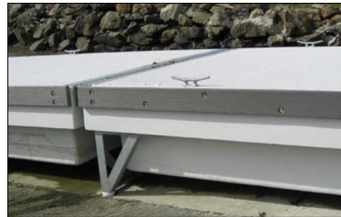
support leg adjacent to float hinge
