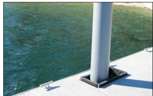
interior pile yoke with raised curb
