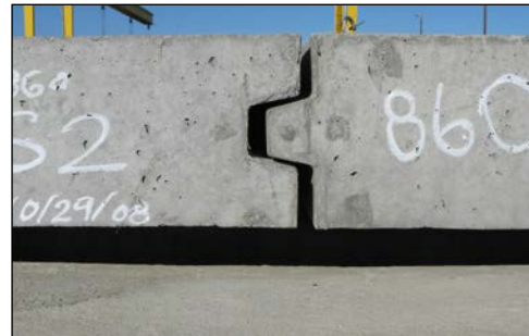
precast concrete panel keys
