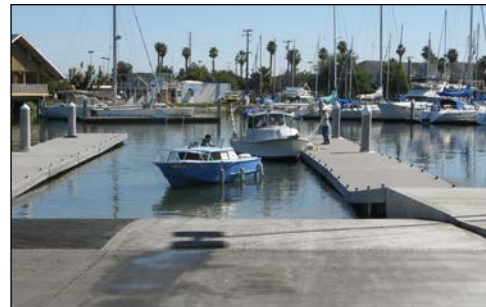
completed precast panel launching ramp
