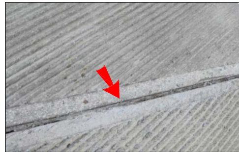
launch ramp construction joint
