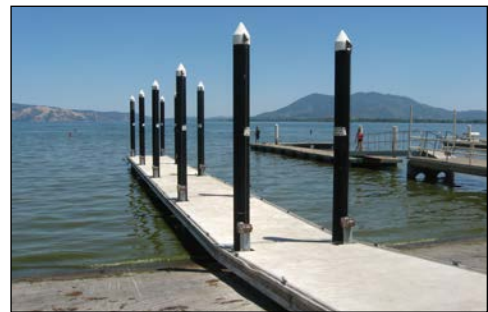
4 sections of suspended platforms
