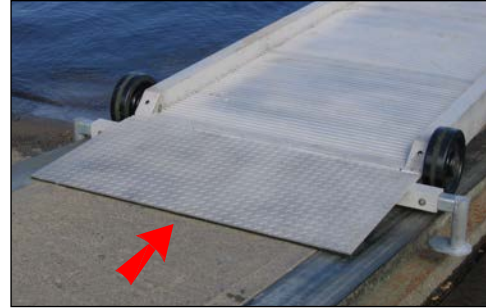
1/2 inch max gangplank leading edge
