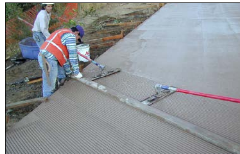
creating diagonal V-grooves in wet concrete
